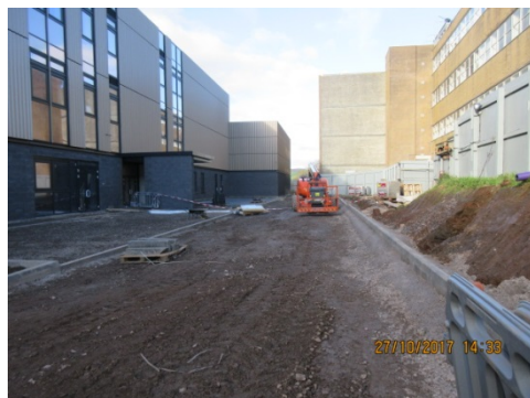
Groundworks continuing on the East elevation in preparation for Tarmac
