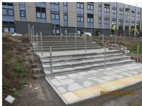
External steps leading to existing grass playing field
