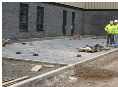
Block paving for disabled person parking bays being installed on the East elevation
