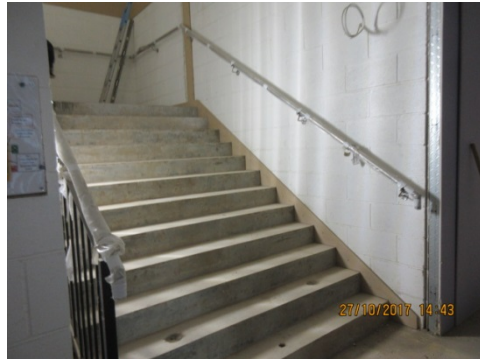
Stringer skirting being installed on stairs
