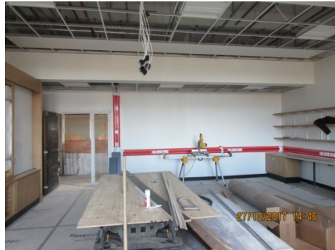
Fitted furniture being progressed on 2nd floor
