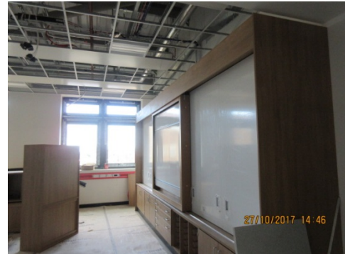
Another classroom nearing completion on 2nd floor
